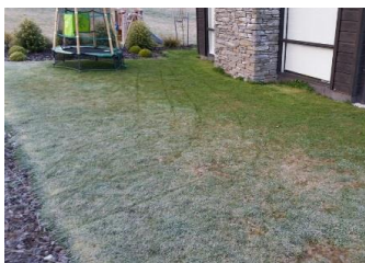
No edge insulation: you're also heating your garden
