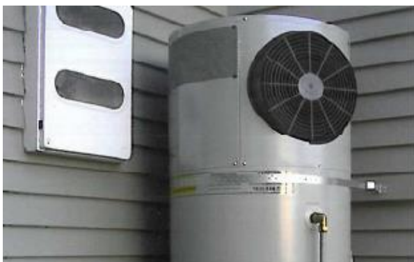
An integral heat pump hot water cylinder is usually sited outside - BRANZ Bulletin 529 Dec 2010
